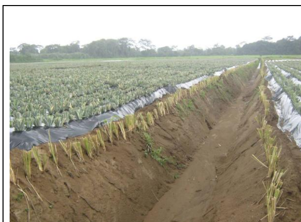
Erosion control: the used of plastic, geotextile and the planting of vetiver grass.
