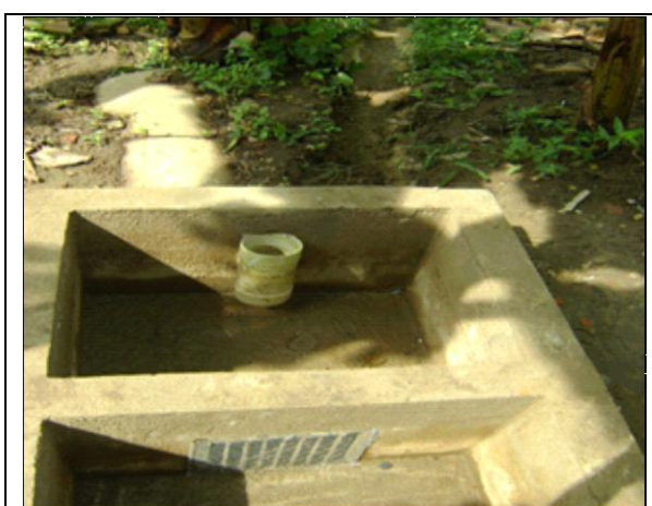
Sediment trap in post-harvest area to prevent runoff.
