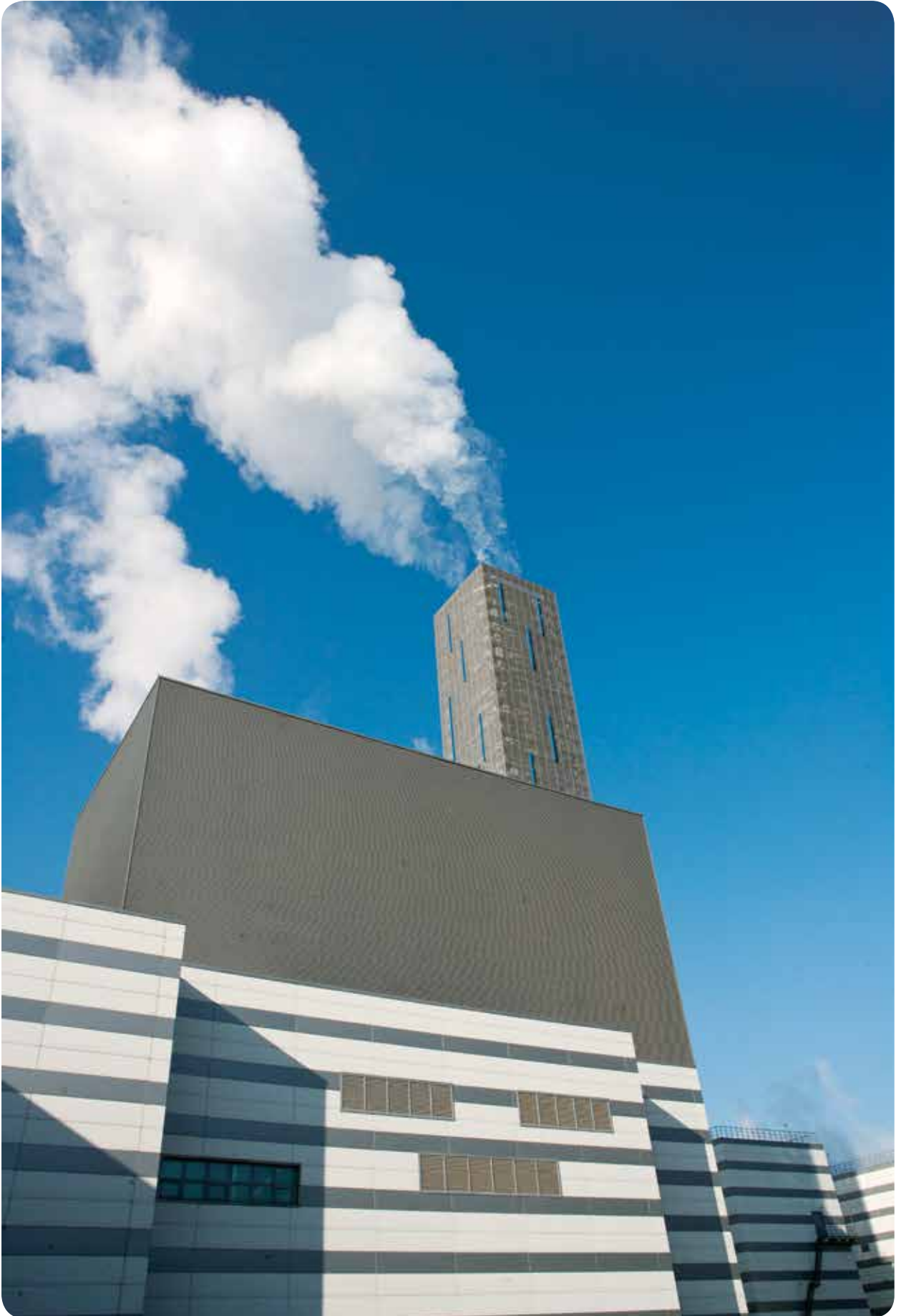
Figure 3.2 A newly built gas-fired power plant in Beijing, 2013
