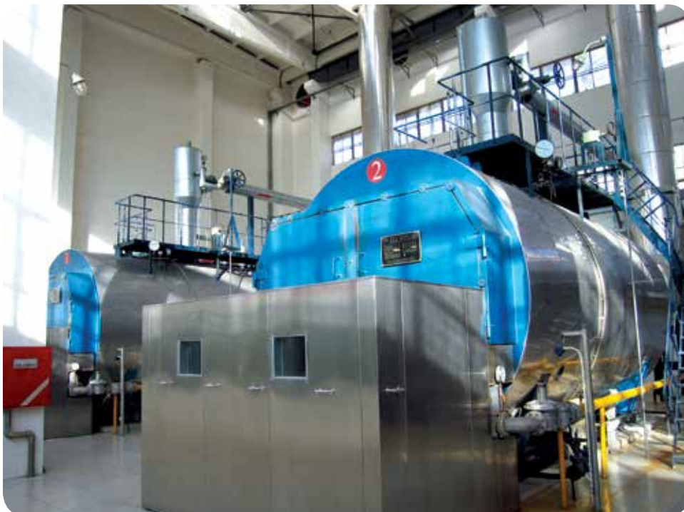
Figure 3.4 Coal-to-clean-energy conversion for boilers
