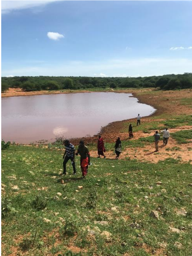
Figure 72: Charco Dam, large and shallow, with livestock access
