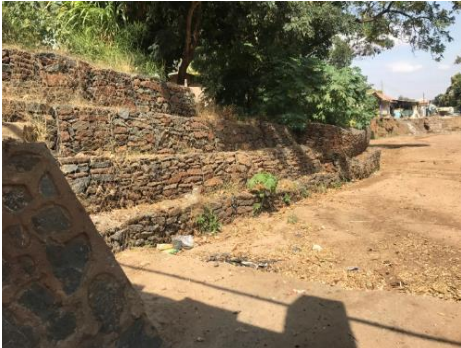
Figure 74: Example of engineering works around Mpwapwa
