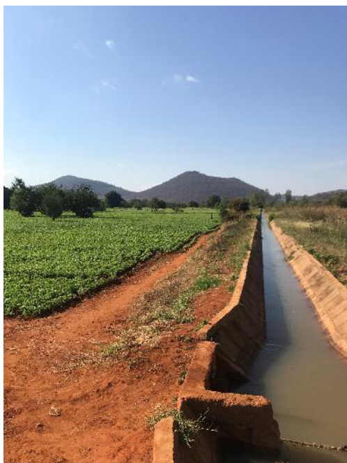
Figure 70: Msagali irrigation scheme
