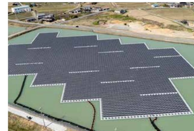
This 2.9 MW floating solar power plant is part of Kyocera's plan to develop 30 such power plants. (Photo: Kyocera)
