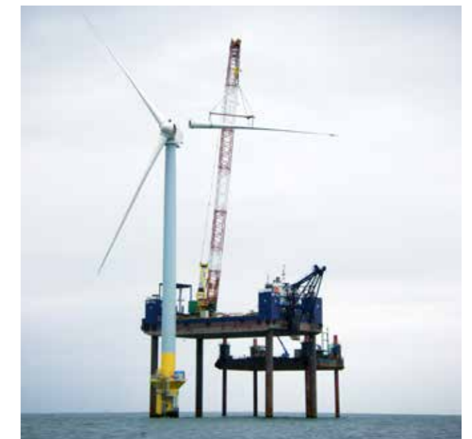
Installation of Japan's first offshore floating wind turbine. (Photo: NEDO, Japan)
