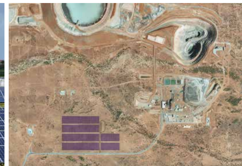
Aerial view of the De Grussa mine solar PV system (Photo: Sandfire Resources)
