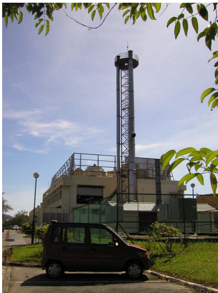
Picture 1: The Medical Waste Incinerator at RIPAS hospital
