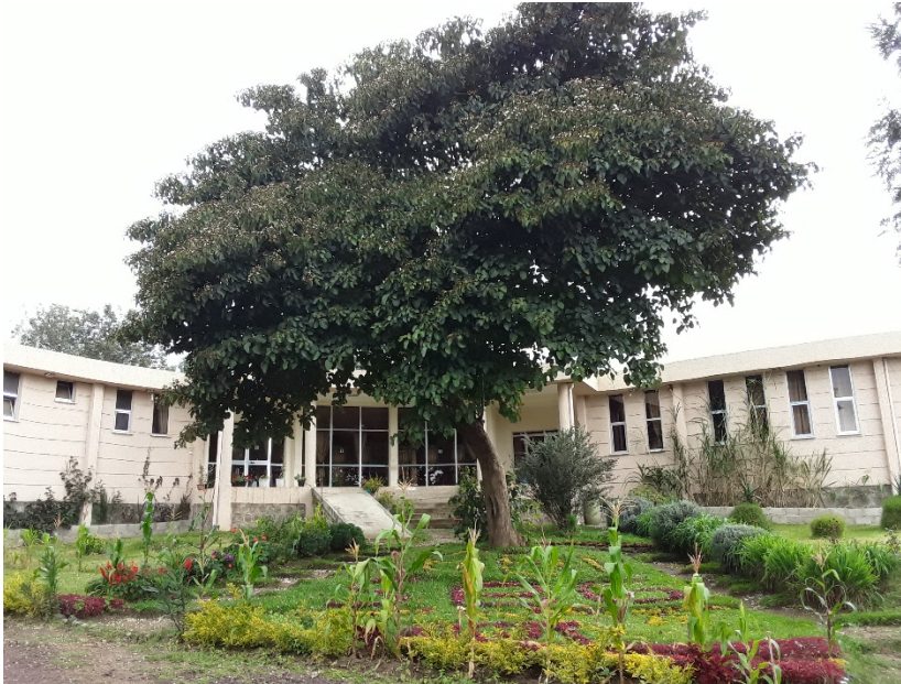
PHOTO 2: THE FACILITY CONSTRUCTED AT THE SHASHEMENE BOTANICAL GARDEN
