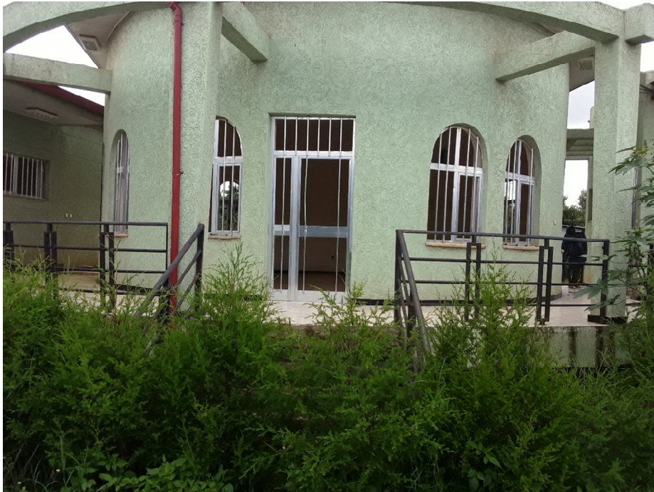
PHOTO 1: THE FACILITY CONSTRUCTED AT THE ZEGIE PILOT SITE
