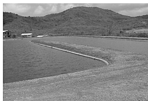
Aerobic Lagoons, St. Lucia (Courtesy CEHI)
