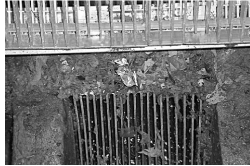
Manually cleaned screens/bar rack St. George's University Grenada (Daniel and Daniel Engineering Inc.)
