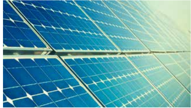
The current solar installation at SBFA Barajii is 90 kW, which represents about 20% of the plant's total energy requirements over a year.
