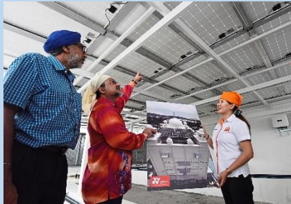
Checking solar panels on top of the gurdwara in Bayan Lepas Photo from TheStar
