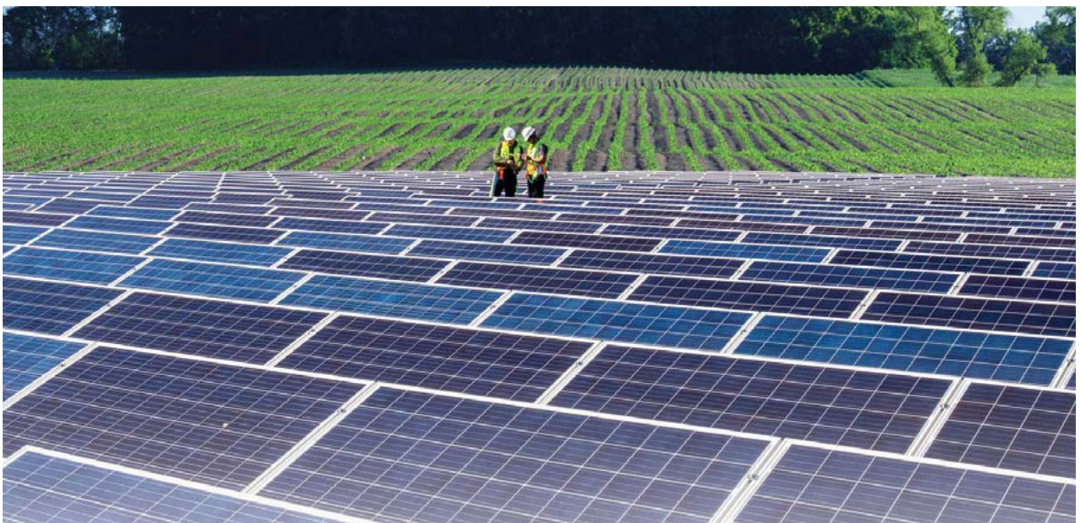
© Specialised Solar Systems
