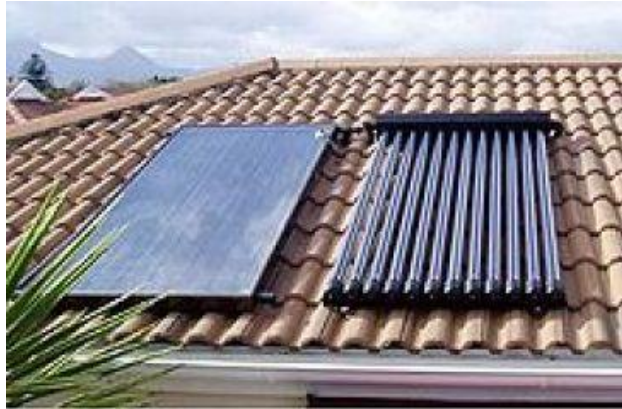
Figure 6: Flat plate and evacuated tube collectors (Northern Lights Solar, 2016)
