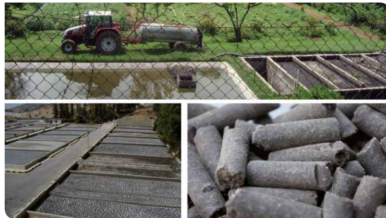
Figure 9. (Above) Settling ponds and drying beds in Uganda (Photo credit: Franz Hollhuber). (Left) Paved sludge drying beds from the Wadi Shueib located in the Salt Valley of Jordan (Photo credit: Calvin College website), (Right) Co-processing of faecal sludge and other urban waste streams to produce fuel pellets, briquettes and crushed fuel in Kampala (Uganda) (Photo credit: Studer et al., 2016).
