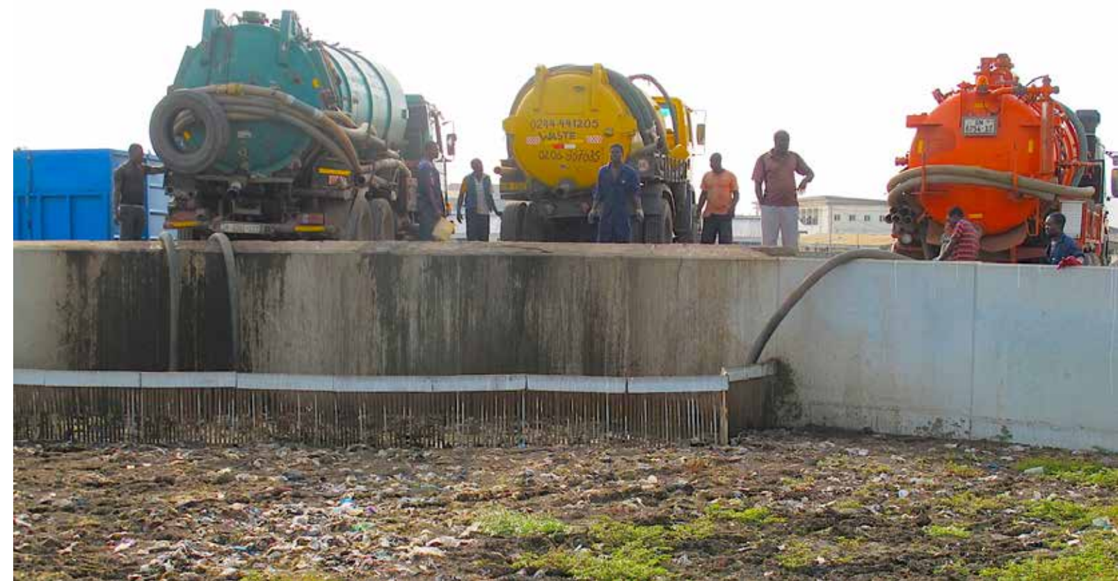
Figure 6. A wastewater treatment facility in Accra Ghana (Photo credit: PATH/R. Wilmouth).
