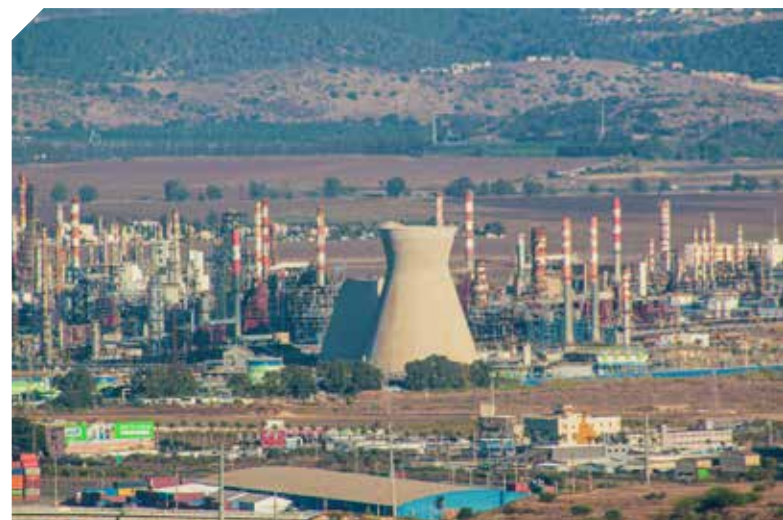
View to cityscape and Industrial Zone with Oil Refineries in Haifa, Israel. Photo credit: © Shutterstock/Max Zalevsky
