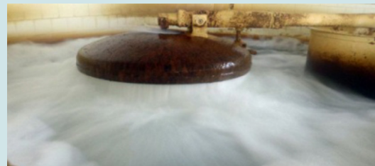
Figure 176 - Water pressure dissipation using a load breaker
