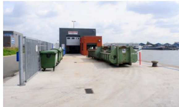
Receptacles for collecting ship-generated waste at a designated and covered area (Photo credits: Peter Van den dries)
