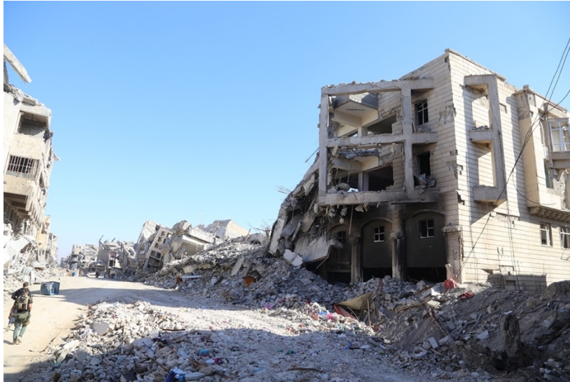
Example of easily accessible rubble on the streets, and 'unreleased' rubble from damaged buildings requiring complex demolition, 2017, UNEP.
