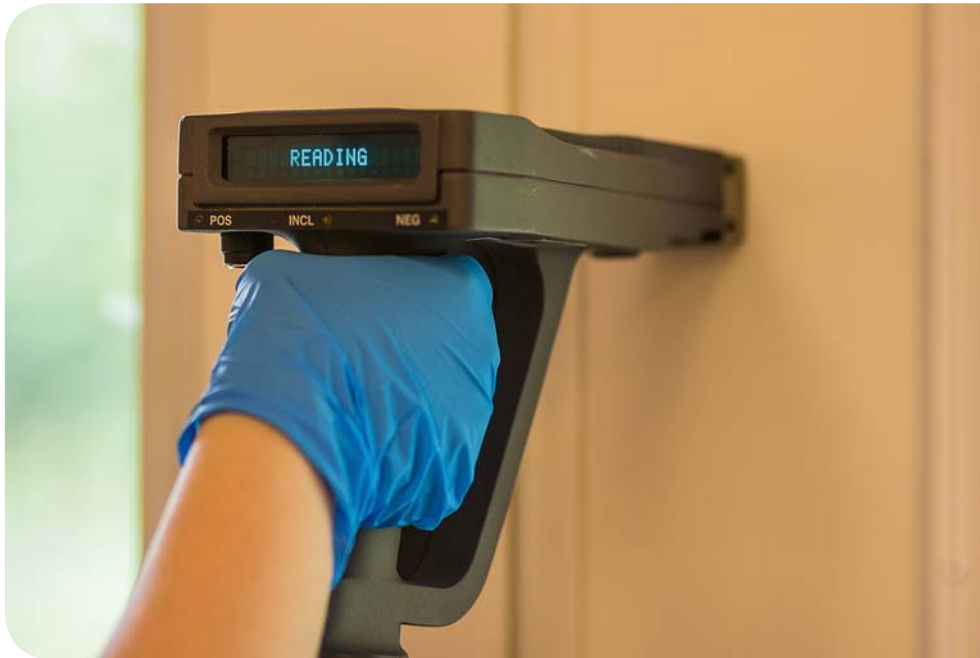
► Figure 4 - Inspection of Lead-based Paint Using and XRF Analyzer
