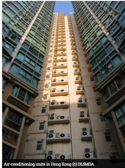
Air-conditioning units in Hong Kong (c) DL5MDA
