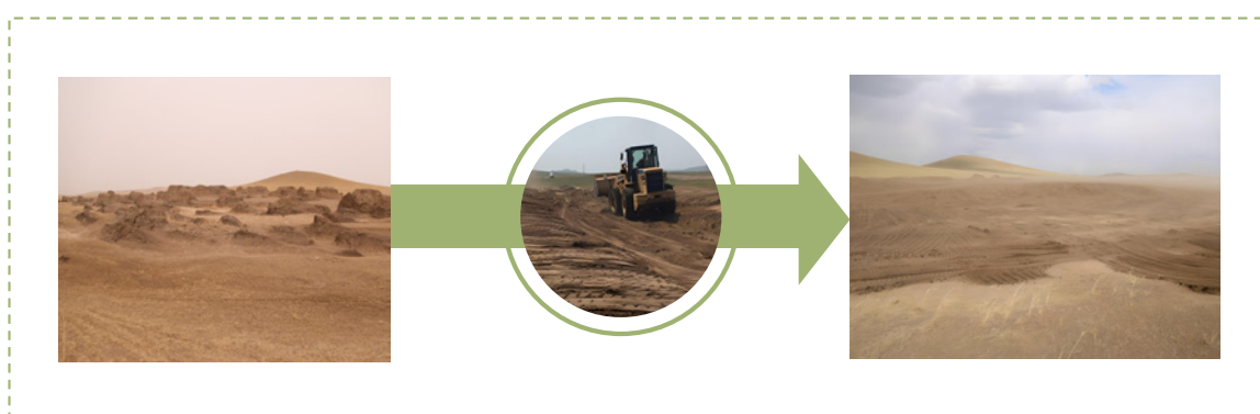
Figure 3.3 Flattening of etching pits using engineering measures (Source: IMGERS, CAS)
