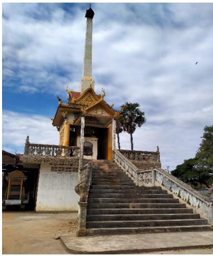
Figure 24: Crematorium in Pagoda at Battambang Province
