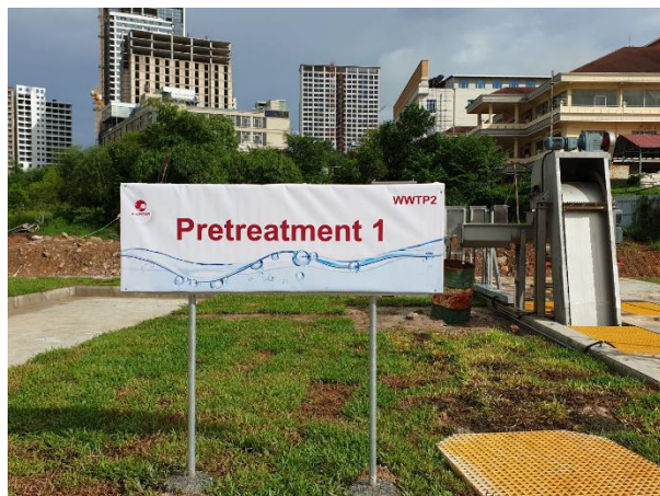
Figure 26: Night soil waste treatment plant in sihanoukville
