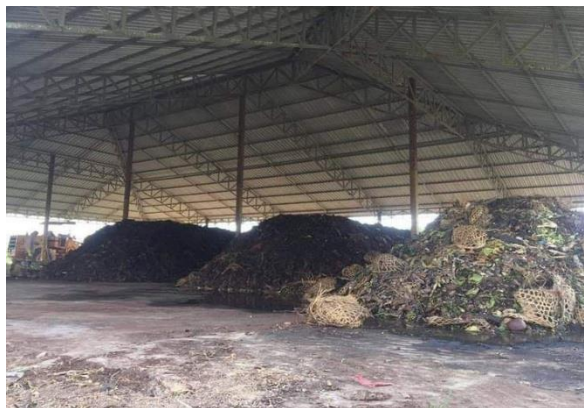
Figure 28: Organic waste collectio for composting, COMPED
