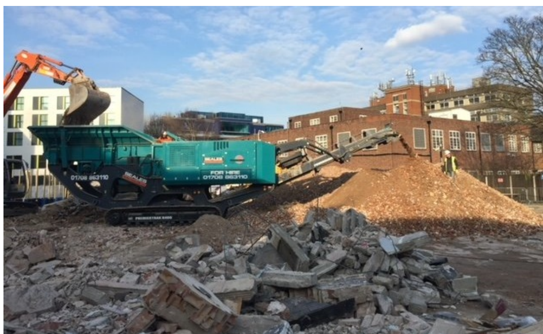
Figure 6:Urban crushing of demolition waste in the UK
