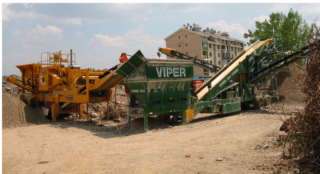
Figure 5:Crushing and screening debris in Gjakova, Kosovo (2001)
