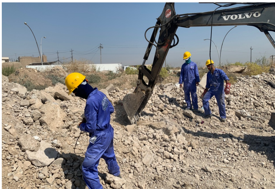
Figure 3: Manual sorting of debris in Iraq with removal of non-recyclables such as plastic, furnishings etc
