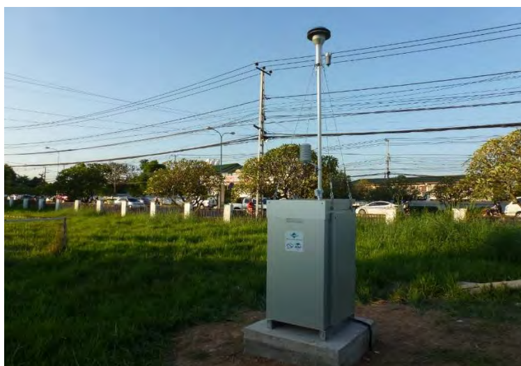
Figure 1.3. Ambient Air Quality Monitoring Station.
