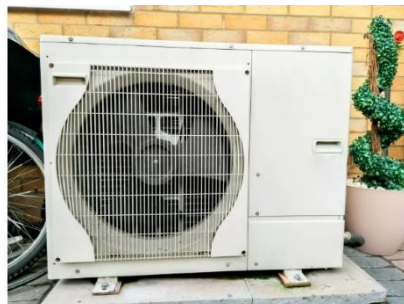
R290 propane refrigerant provides alternative to F-gas refrigerants (Image credit: Getty)
