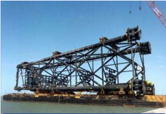
Offshore transportation by tow barge
