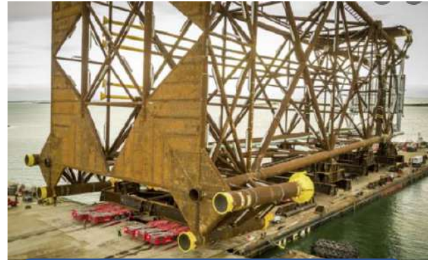
SPMT Transfer to laydown area
