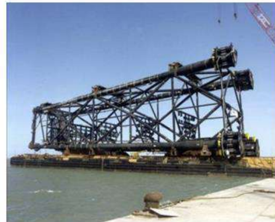
Transportation of WHP's topside and jacket to onshore licensed dismantling facility
