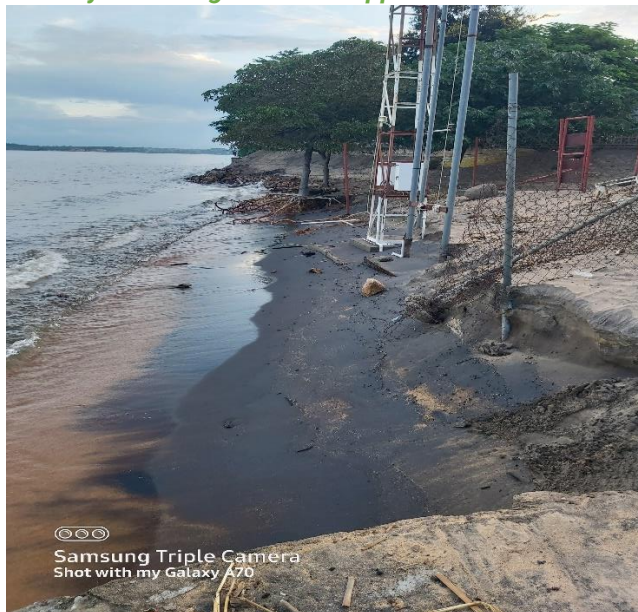
Figure 3: Partially Submerged EADN-Supported Weather Station in Senga Bay
