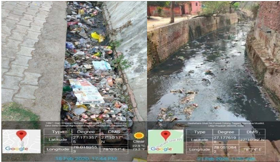
Figure A1.45: Open Drain was Clogged Due to Plastic Waste
