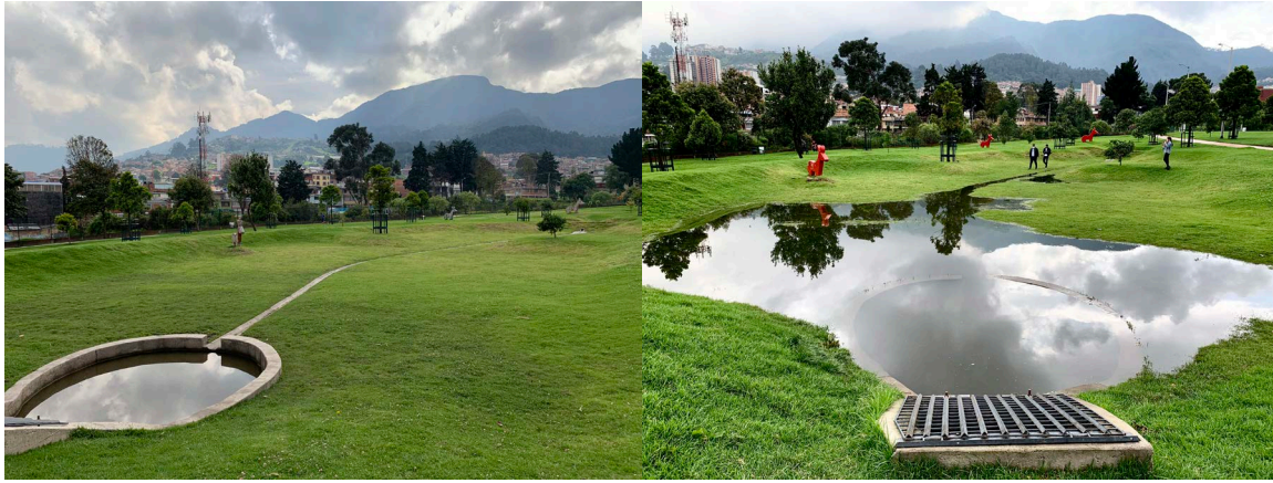
Figure 5.1: SUDS (extended drainage dry basin) in the Metropolitano San Cristóbal Sur Park, Bogotá, Colombia.
