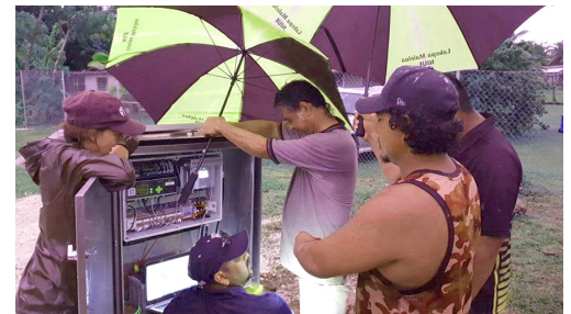
Installation of an Automatic Weather Station in Niue
