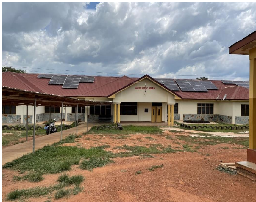
Figure 10: Photo from St. Marys Hospital, Pediatric Ward, with installations of solar PV systems on the roof of hospital buildings in Ghana (Photo: Yamini Jain, May 2023)
