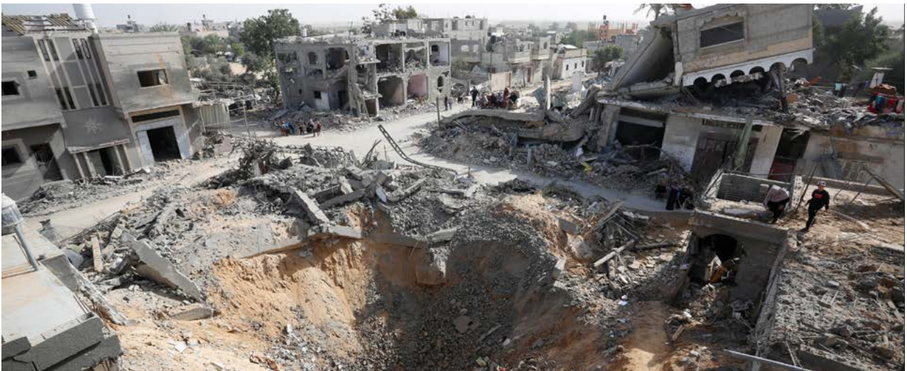
26 November 2023, collapsed buildings and scenes of destruction in Khan Yunis © UNRWA Photo by Ashraf Amra
