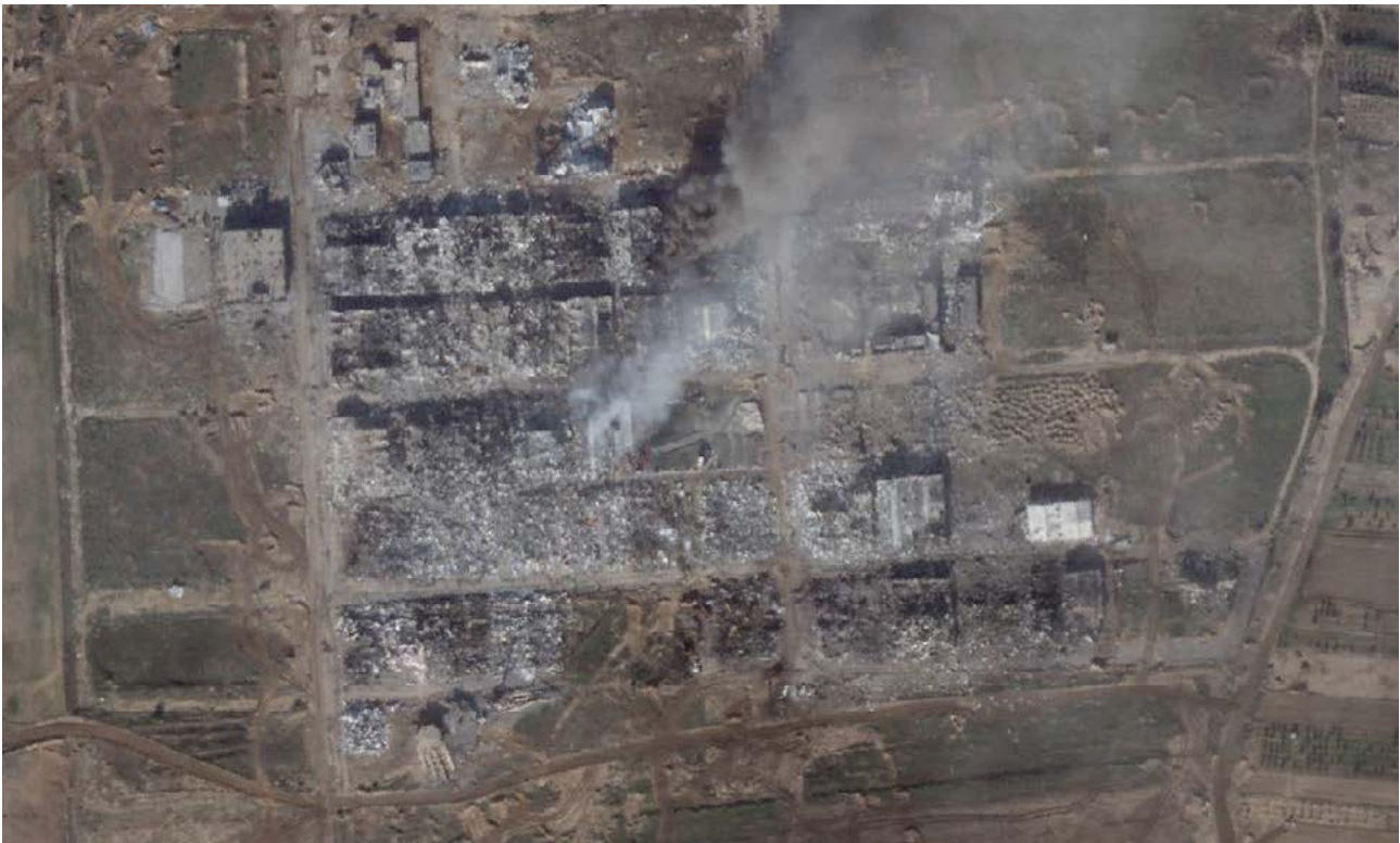
Figure 5: A satellite image taken on 16 December 2023 shows the almost complete destruction of the Gaza Industrial Zone. Source: World Bank.
