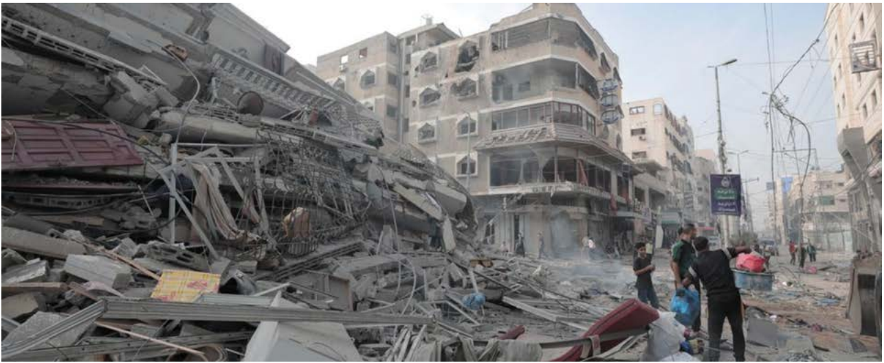
A building collapsed into the street in Gaza. © UNRWA/Mohammed Hinnawi
