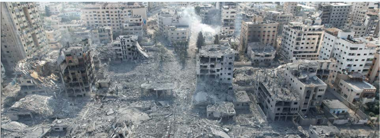
October 2023, aerial view of collapsed buildings and destruction in the Gaza Strip © United Nations Photo
