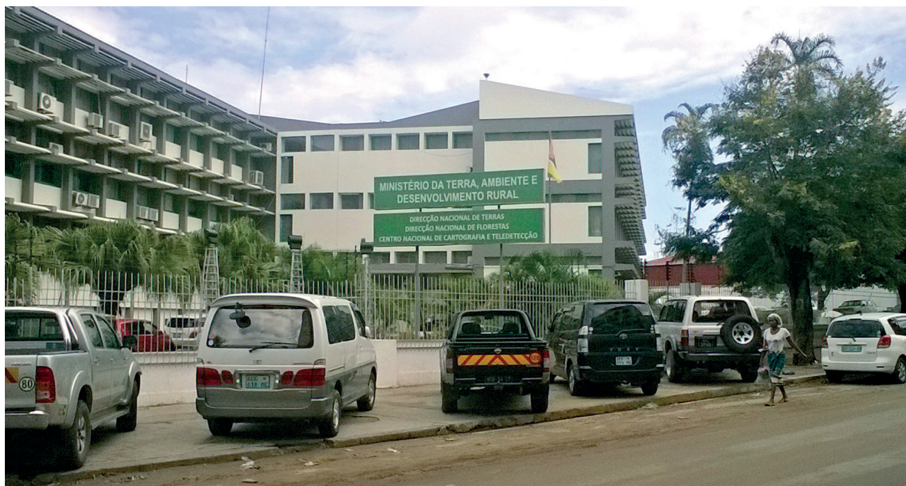
FIGURE 8. MITADER headquarters, Avenida Josina Machel, Maputo, one of eight sets of offices, housing three other entities (related to cadastral services and mapping, and forestry).
