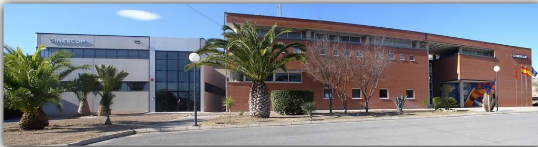
Figure 1. INESCOP's Headquarters in Spain
