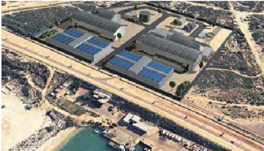
Figure 12: Ashkelon 320,000 m 3 /day desalination plant in Israel. The largest desalination facility on the Mediterranean Sea.
