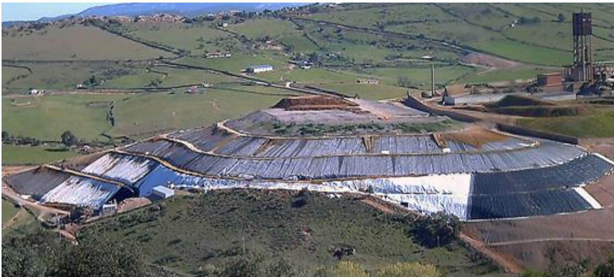
CERCO DE SAN TEODORO SLAG HEAP MARCH 2007
