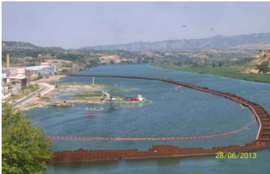
Dredging activities inside the sheet piling
