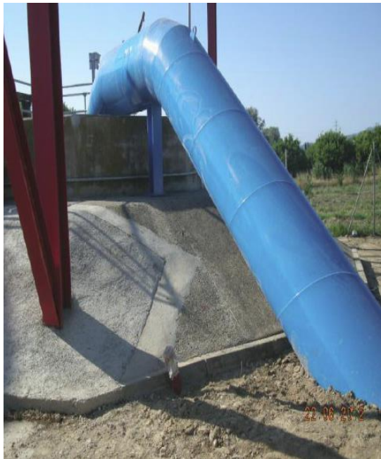
One of the wells constructed for drinking water supply to downstream towns in case of emergency
