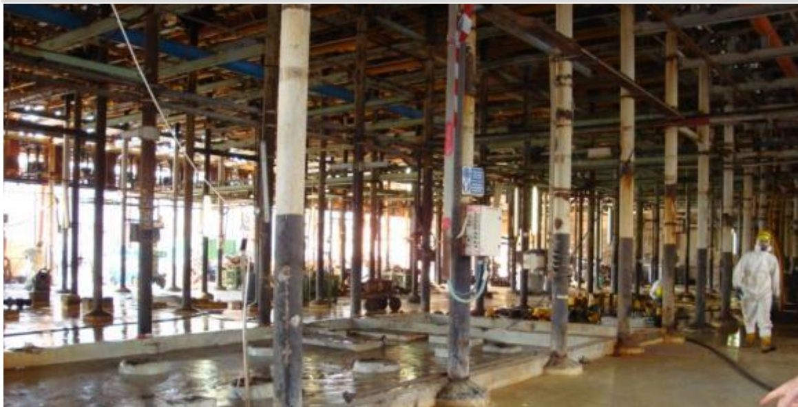
Floor of cell room regularly washed down
