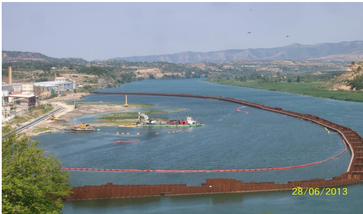
Dredging activities inside the sheet piling
