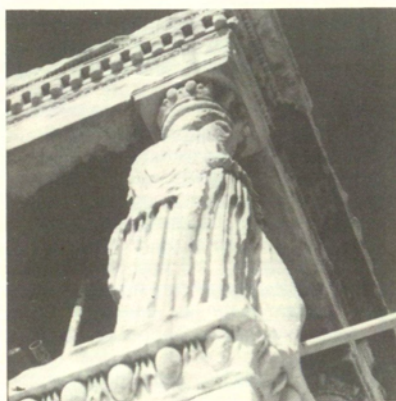
Air pollution in Athens has created several problems; one of them is the slow erosion of the white marble, the material used by the ancient Greeks in the construction of their temples as well as the creation of works of art; one of the famous Caryatides, shown here in its present condition, is a typical example. SO 2 , the main cause of this erosion, has been radically reduced over the last decade.
