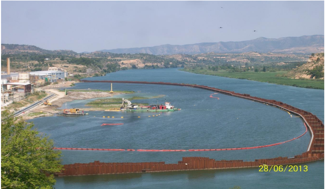
Dredging activities inside the sheet piling
