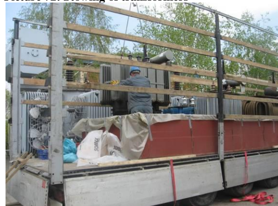
Picture 72: Stowing of transformers
