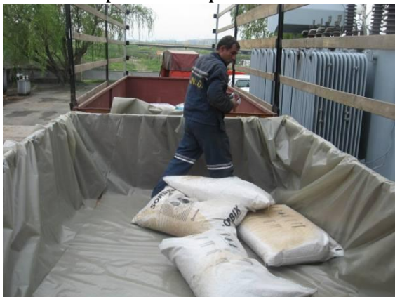
Picture 69: Preparation: transportation of PCB transformer
