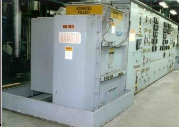
Picture 39: Retention system made from steel
