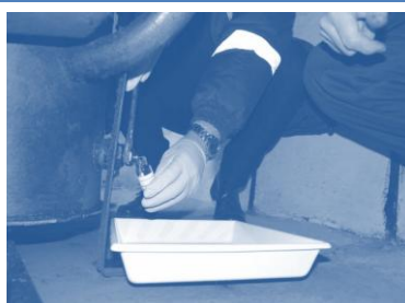
Place drip tray under drain tap, wearing gloves and goggles
