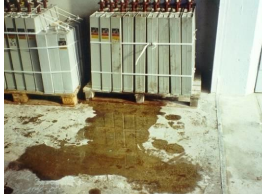
Picture 85: Bad example II (no tip trays)
