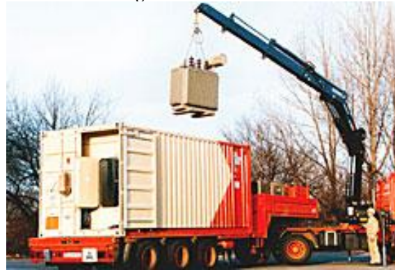
Picture 100: Loading of transformers
