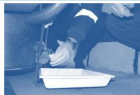
Place drip tray under drain tap, wearing gloves and goggles
