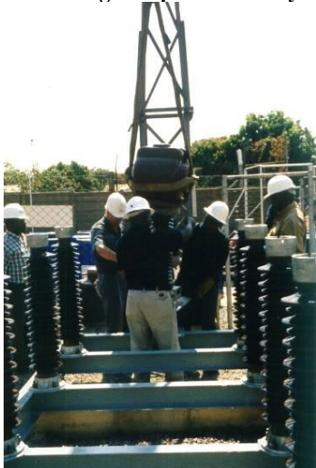
Picture 55: Dismantling of capacitor battery
