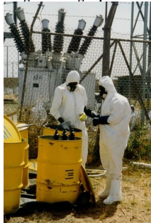
Picture 58: Packing of leaking caps into UN drums
