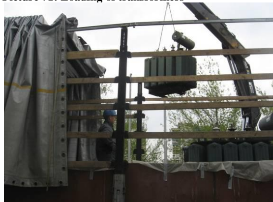
Picture 71: Loading of transformers
