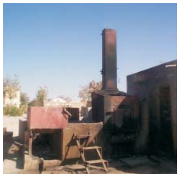
Incinerator at Mirwais Civilian Hospital, Kandahar
