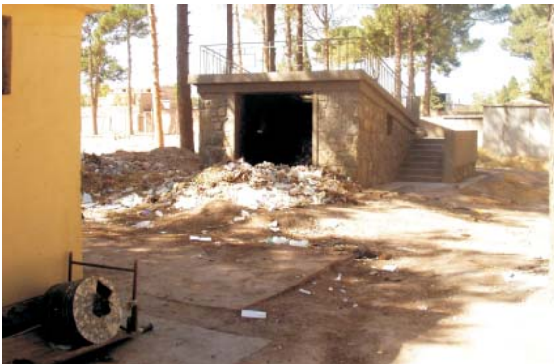
Collection point for medical waste at Herat Region Hospital
