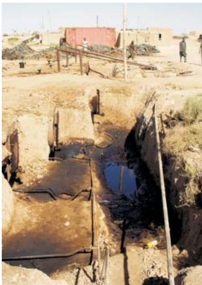
Boilers leaking crude oil onto the ground at Shiburghan
