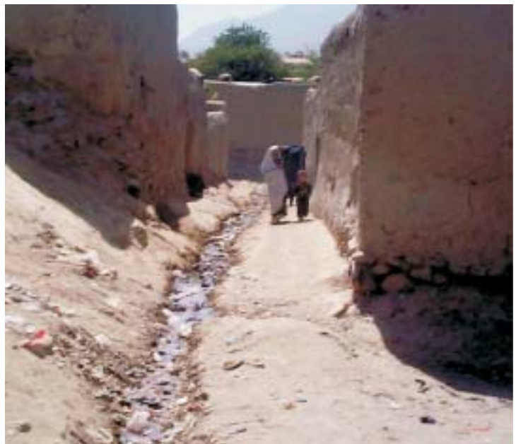
Open sewer in District 5 of Kabul
