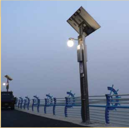
Lightron Lighting & Advancement
