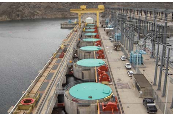
Covered hydro turbine generators on Wells Dam, Columbia River, Washington. Photo credit: Kevin Davis.
