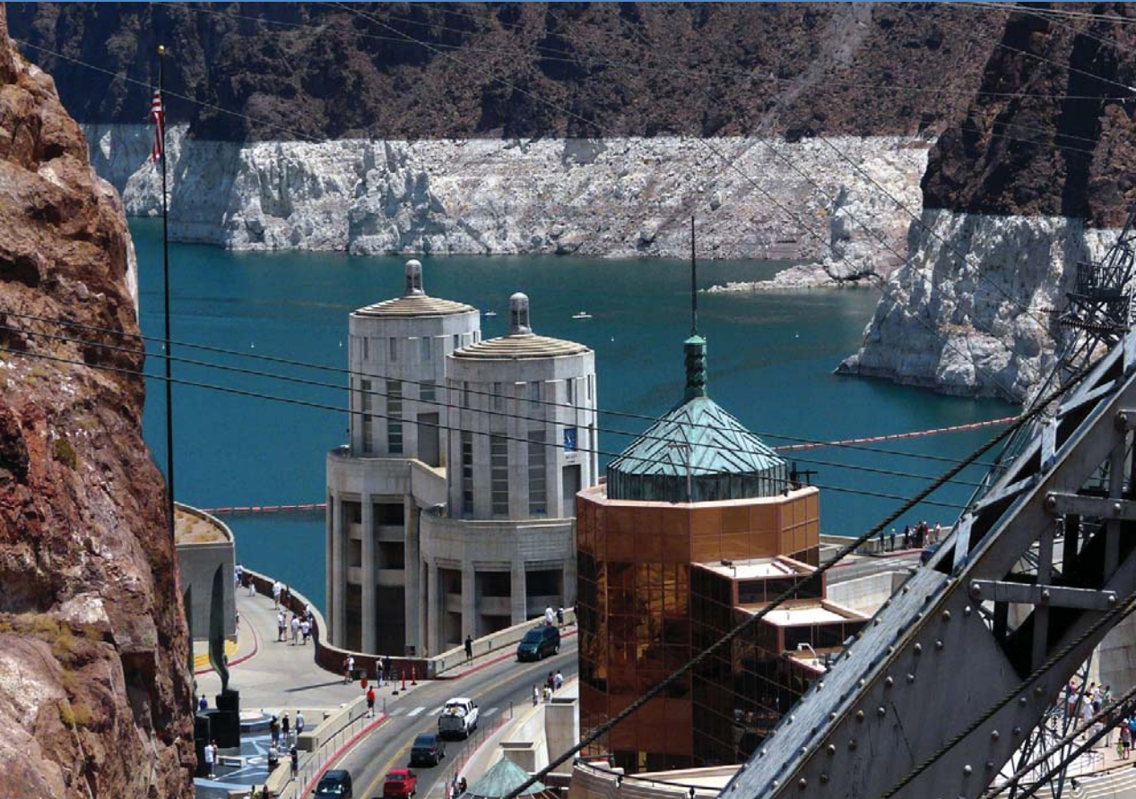
Hoover Dam, on the Colorado River between the states of Nevada and Arizona. Photo credit: Terrence E. Davis.
