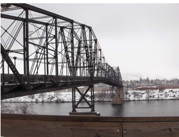
(top) Potatoes under irrigation, with wheat fields in the background, Idaho. Photo credit: Terrence E. Davis. The century-old Wenatchee Bridge, the first highway bridge over the Columbia River, still carries irrigation water in two pipelines to apple orchards in East Wenatchee, Washington. Photo credit: Kevin Davis.
