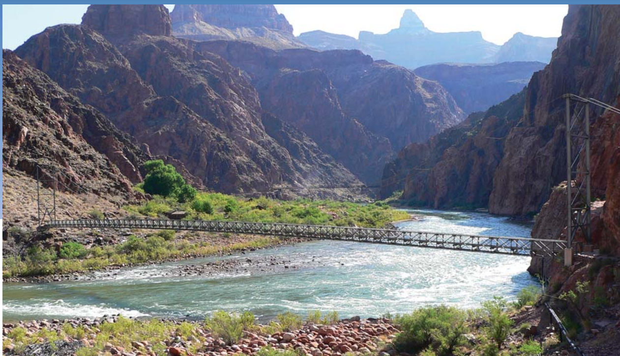
Silver Bridge over the Colorado River; Black Bridge in the distance. The Silver Bridge supports the trans-canyon waterline, which brings water from Roaring Springs to the pumping station at Indian Gardens and supplies water for Grand Canyon National Park. Photo credit: Terrence E. Davis.
