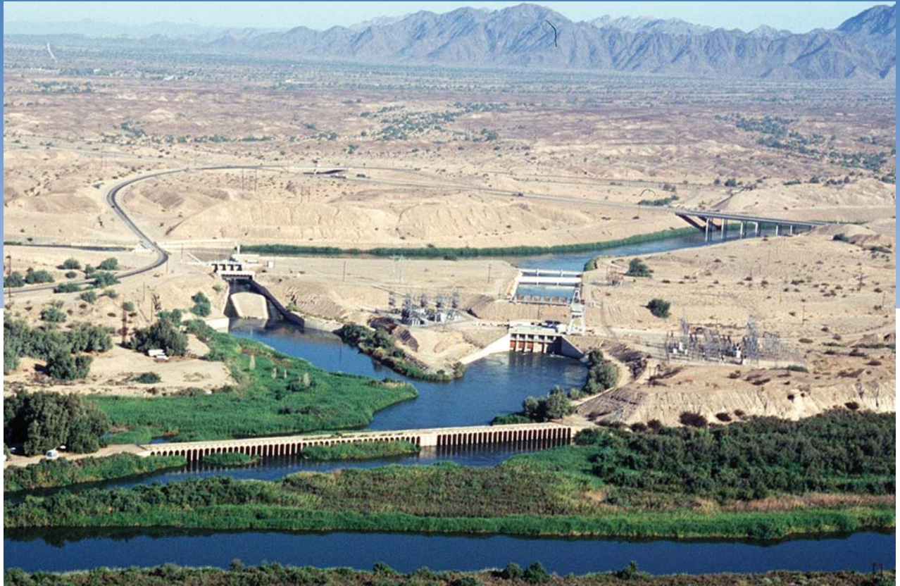
Siphon Drop Power Plant on the Yuma Canal (offshoot of the All American Canal). Photo credit: Andy Pernick, courtesy of U.S. Bureau of Reclamation.
