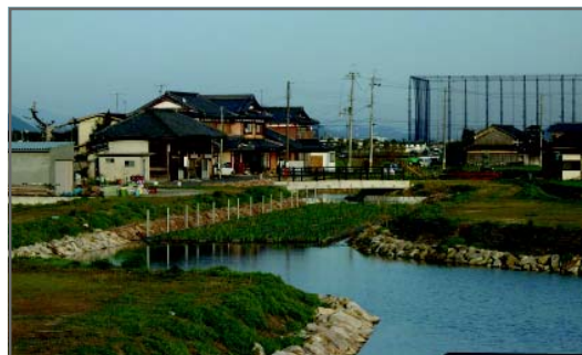
Fig. 10.2 Constructed wetland for surface runoff from arable land, Japan (photo: V. Santiago-Fandino)
