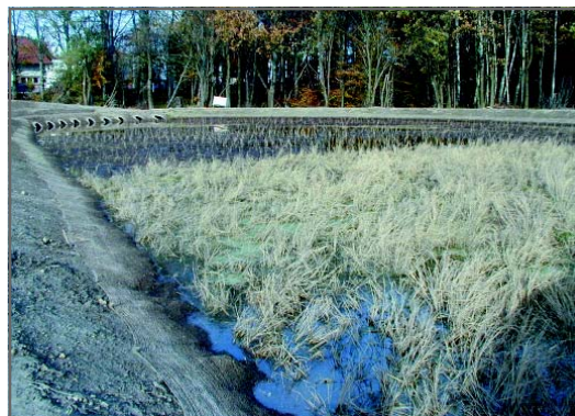
Fig. 10.1 Constructed wetland for storm water Karls-Einbau Project Company (photo: EKON Polska Biologia Inzynieryjna Sp. z o.o.)
