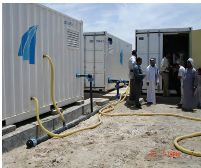
Figure 7 Water treatment facility during construction
