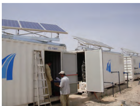
Figure 10 Photovoltaic system installation at Al-Ghreej water treatment plant
