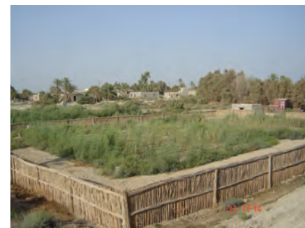
Figure 14 Constructed wetland facility for sanitation pilot project at Al-Chibayish
