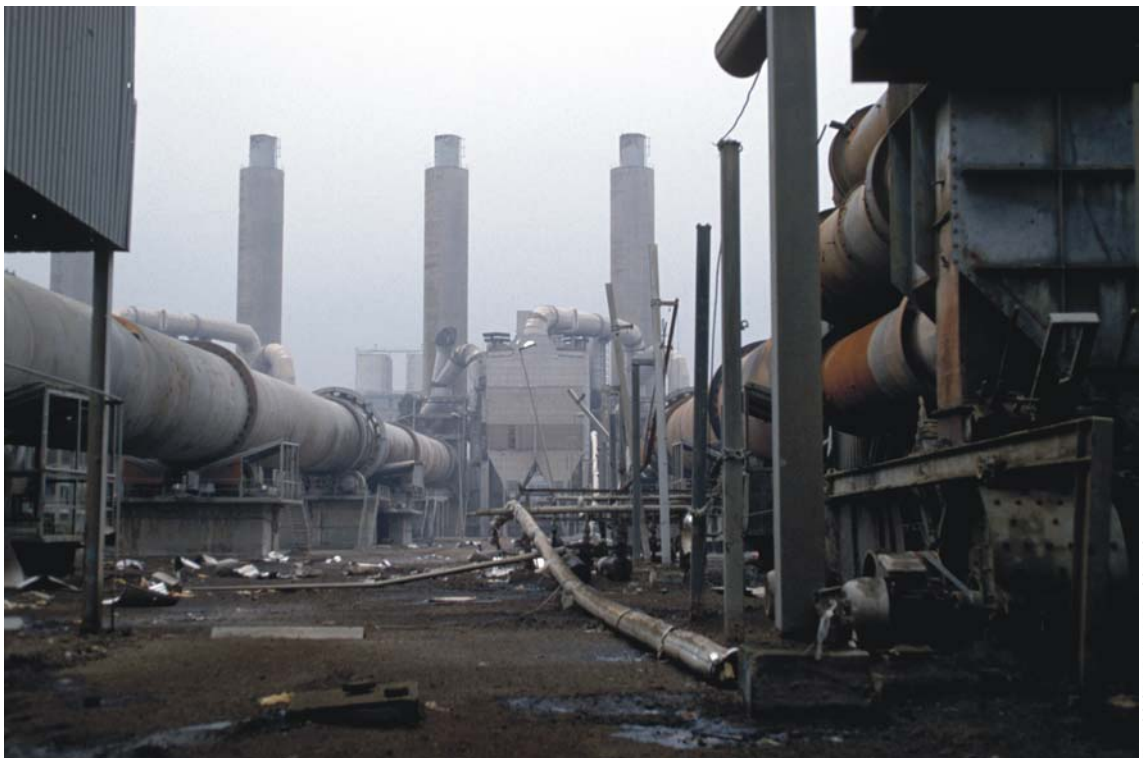
Iraq's Dora oil refinery, bombed during the 1991 Gulf War
