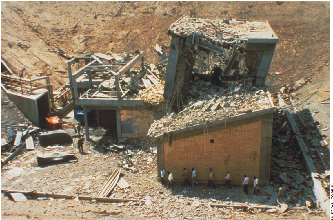
Destroyed chemical weapons bunker at Al Muthanna
