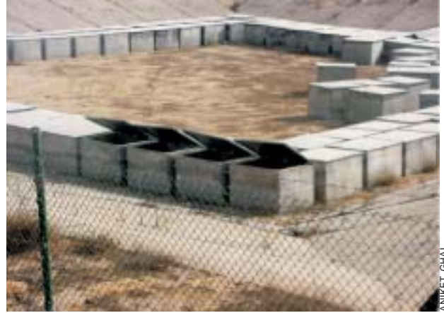
Hazardous waste temporary storage facility in Gaza
