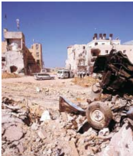
Damage sustained to the headquarters in Ramallah of His Excellency Yasser Arafat, President of the Palestinian Authority
