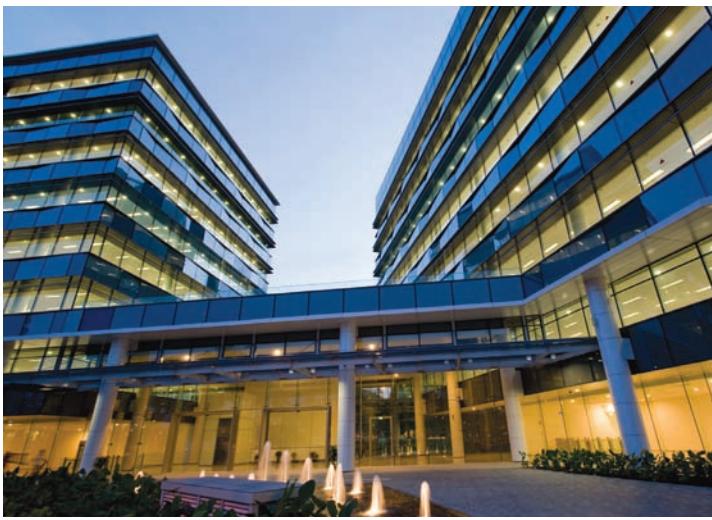
Forty customised large sized 152 Wp amorphous silicon thin-film Building Integrated Photovoltaic (BIPV) Panels have been installed on Tampines Grande's facade across an area of 140 square metres to give an output of 6 kWp. The customised BIPV panels form part of the facade cladding, replacing conventional glass that would otherwise have been used.
