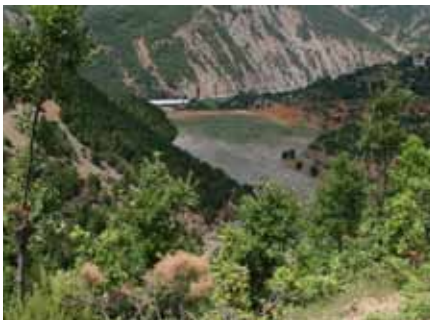
View on Reps tailings dam
