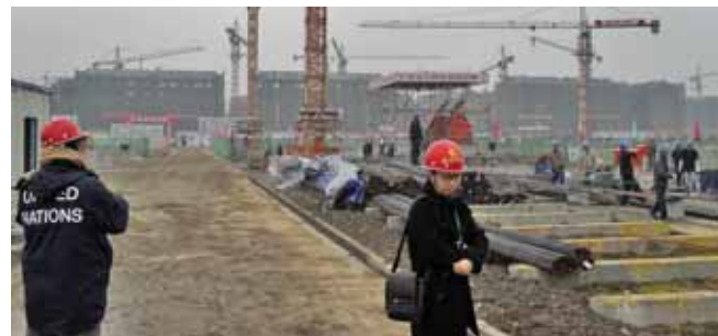
The ongoing reconstruction process integrates environmental and disaster reduction considerations
