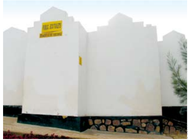
Public ecological toilets in Kigali city center
