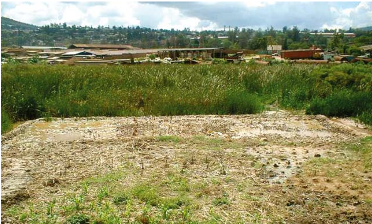
Soil compaction in wetlands for construction affects their ecological properties as it is the case in Gikondo-Nyabugogo wetland
