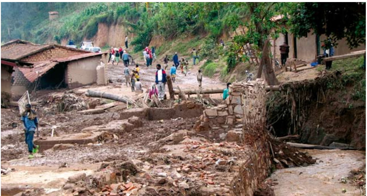
Effects of floods in Rulindo District Northern Province in 2006
