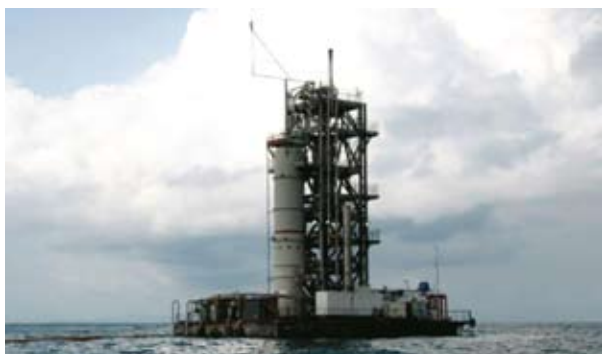
Methane gas power plant in Lake Kivu
