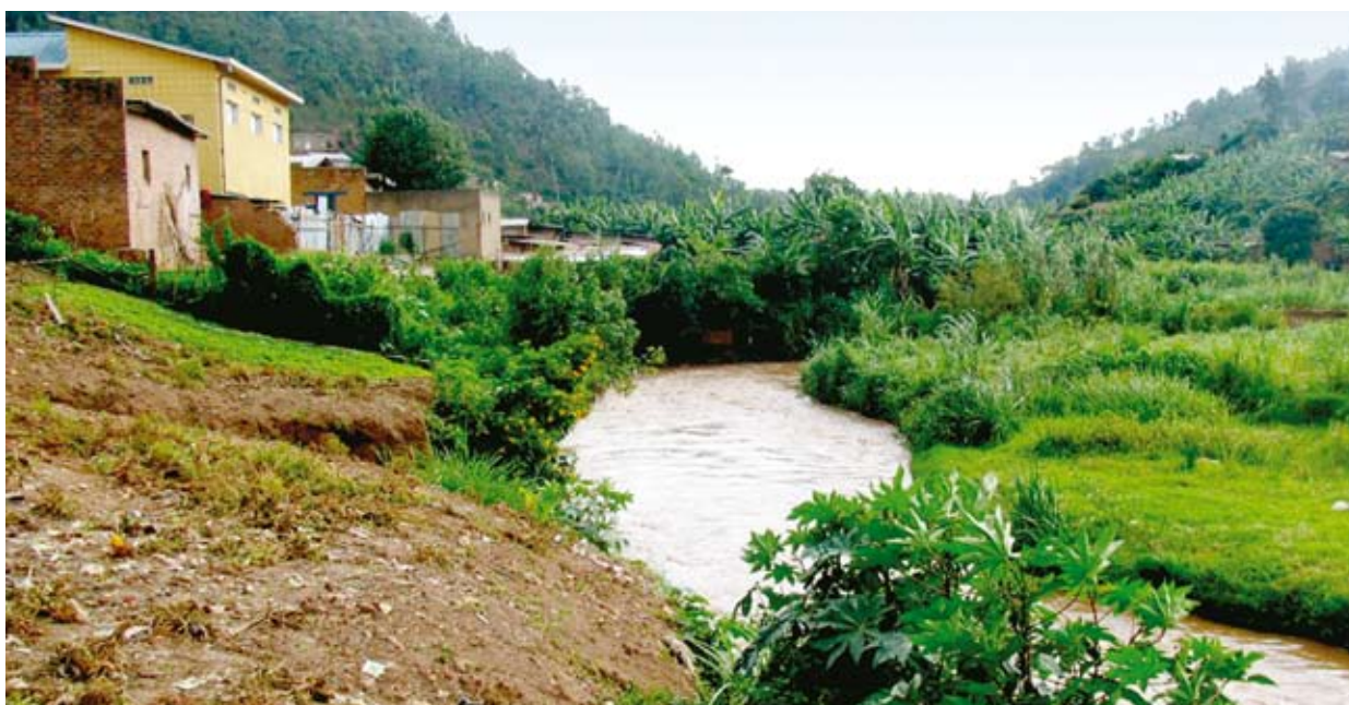
Construction in a wetland at the banks of Nyabugogo River in Kigali
