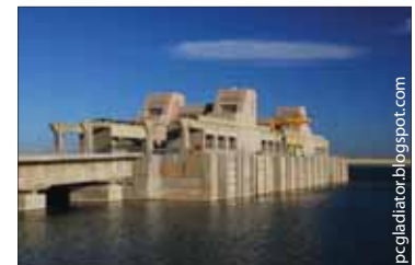
The Mubarak Pumping Station pumps water from Lake Nasser into the irrigation channels
