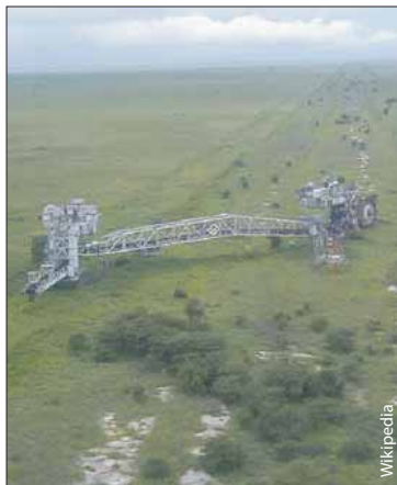
Construction of the canal ended in 1983 and the digger has remained here since
