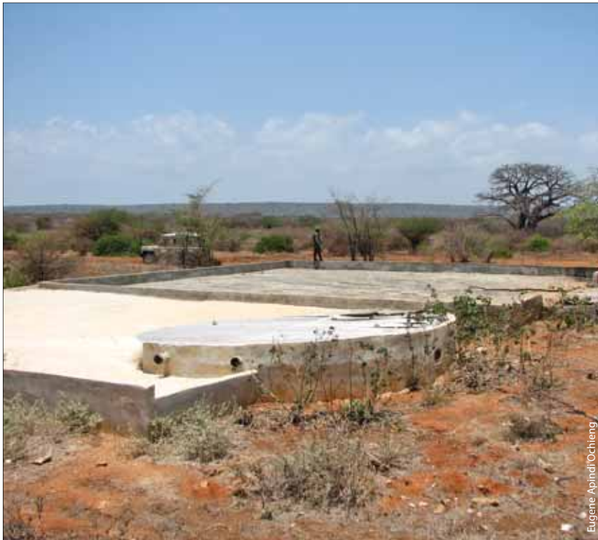
This concrete slab in northeastern Kenya collects rainfall and diverts it into an underground storage tank for later use
