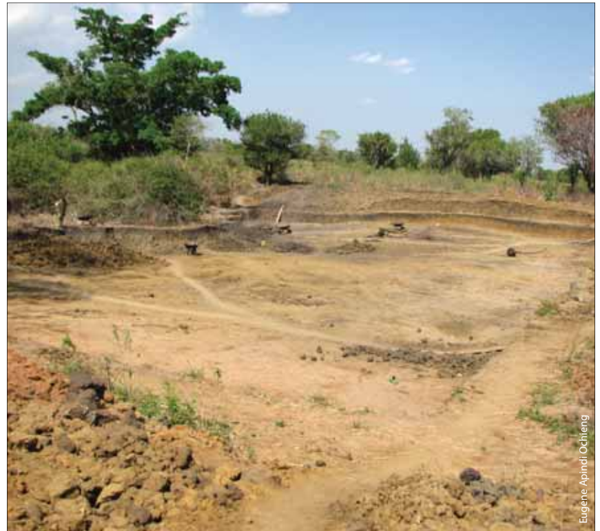
Water harvesting pond under construction in Lamu District, Kenya
